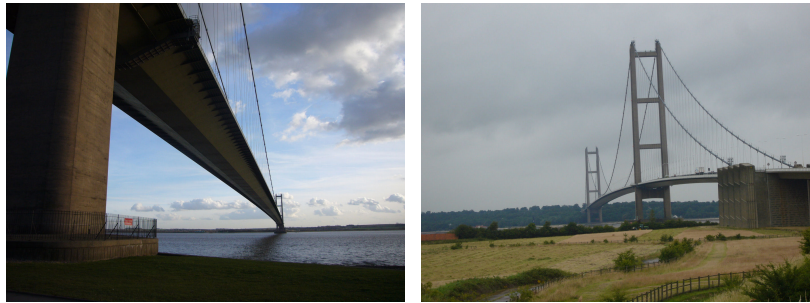
Fig. 4 Views of Humber Bridge from North and South.
