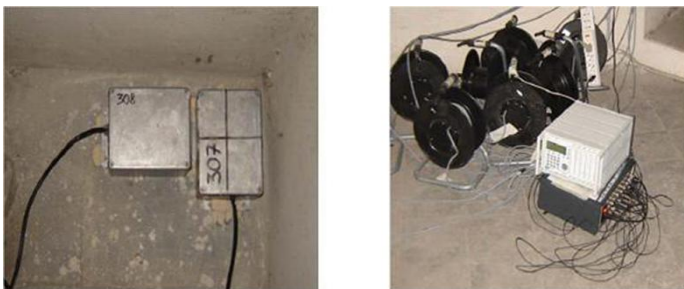
Fig. 2. Accelerometers and acquisition board used for the tests.
