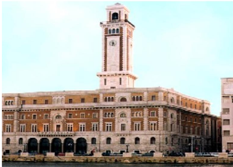
Fig. 1. View of the Provincial Administration Building of Bari (a) and of the investigated tower (b)
